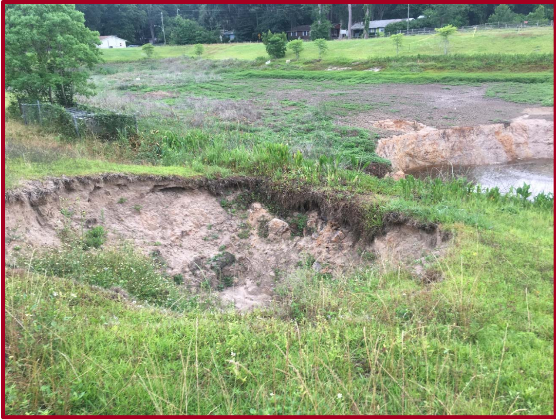
FIGURE 3C: PHOTOGRAPH OF EXISTING SITE CONDITIONS NEAR SOIL BORING VB-1 (FACING EAST)
