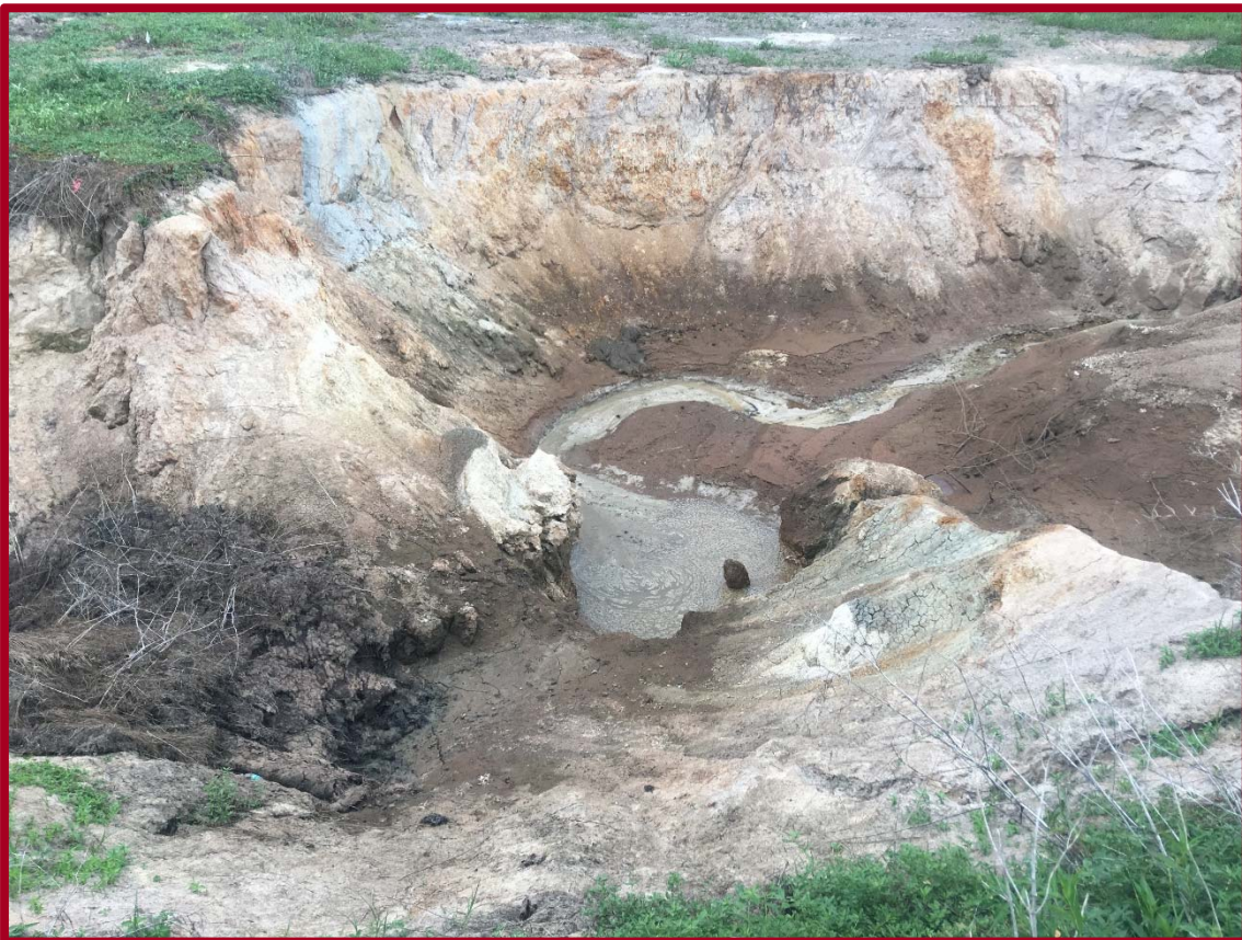
FIGURE 3B: PHOTOGRAPH OF EXISTING SITE CONDITIONS NEAR SOIL BORING VB-11 (FACING EAST)
